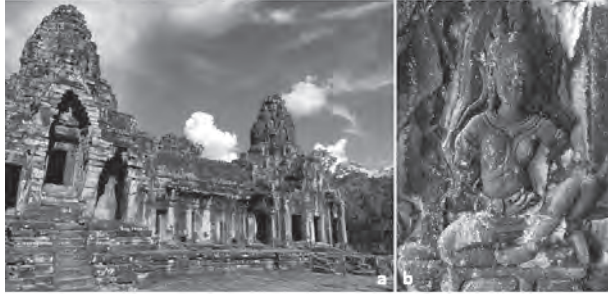
Figure 1 Microbial colonization, colors and deterioration of sandstone wall at the Angkor Bayon temple gallery
